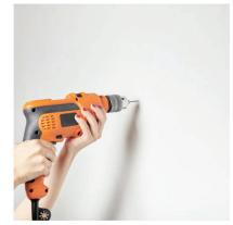
DRILL HOLES FOR WALL ANCHORS USING 5/16" DRILL BIT
